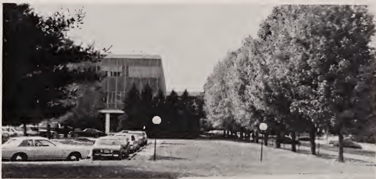
AVCO carried the M.D.C. sewer from the Woburn line and moved into Town in 1959
